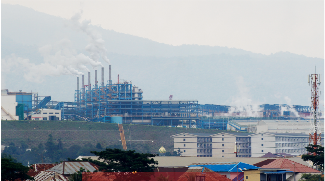
Figure 11. Emissions from Coal-Fired Power Plants
